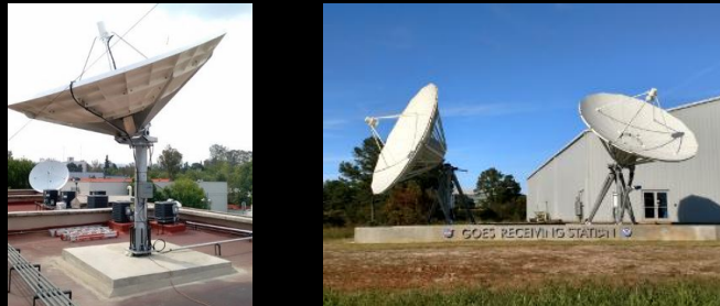
Typical GRB Receiving Antennas
