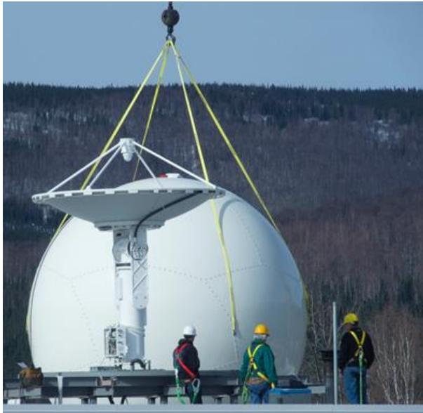
Stemming from collaborative efforts between NOAA via the JPSS Proving Ground and Risk Reduction (PGRR) Program, the NWS, and GINA, a new 3.0 meter X, L, and S band antenna from Orbital Systems was installed in April 2015 at FCDAS. This installation ran concurrent with NWS communication upgrades.
